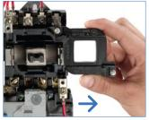
No need to remove any wiring!
