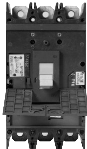
Fig. 3.2 View of SG Frame breaker with accessory pouches open, accessories displayed
