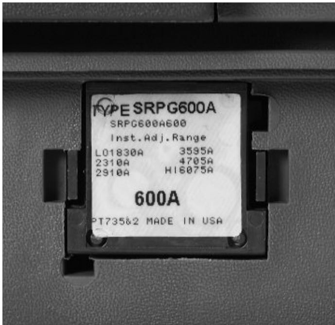
Fig. 7.1 Rating plug label
